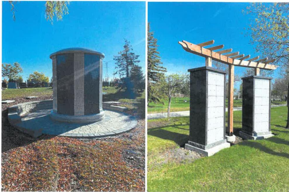
Dome Columbarium Structure (72 niches)
